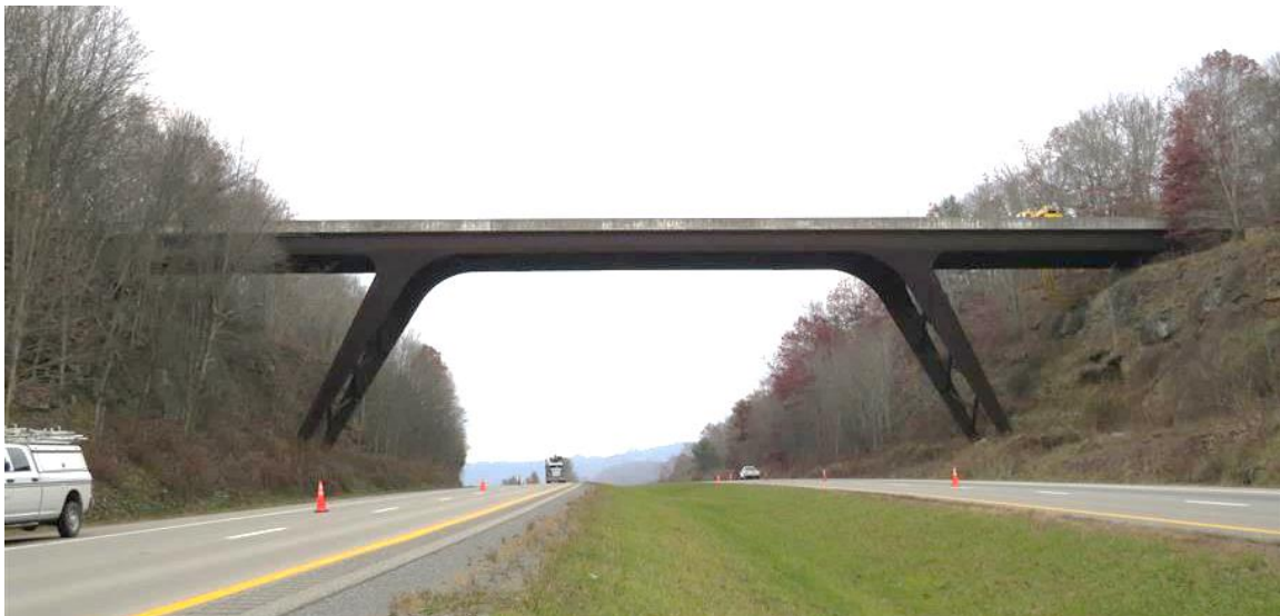
Figure 35. The Loudermilk Road Bridge (BARS13A122) inspection photo, 2023.
