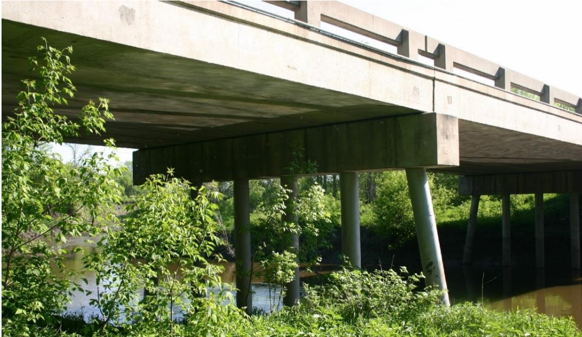
Figure 3. Example of a prestressed-concrete box beam structure. Mead & Hunt photograph.
