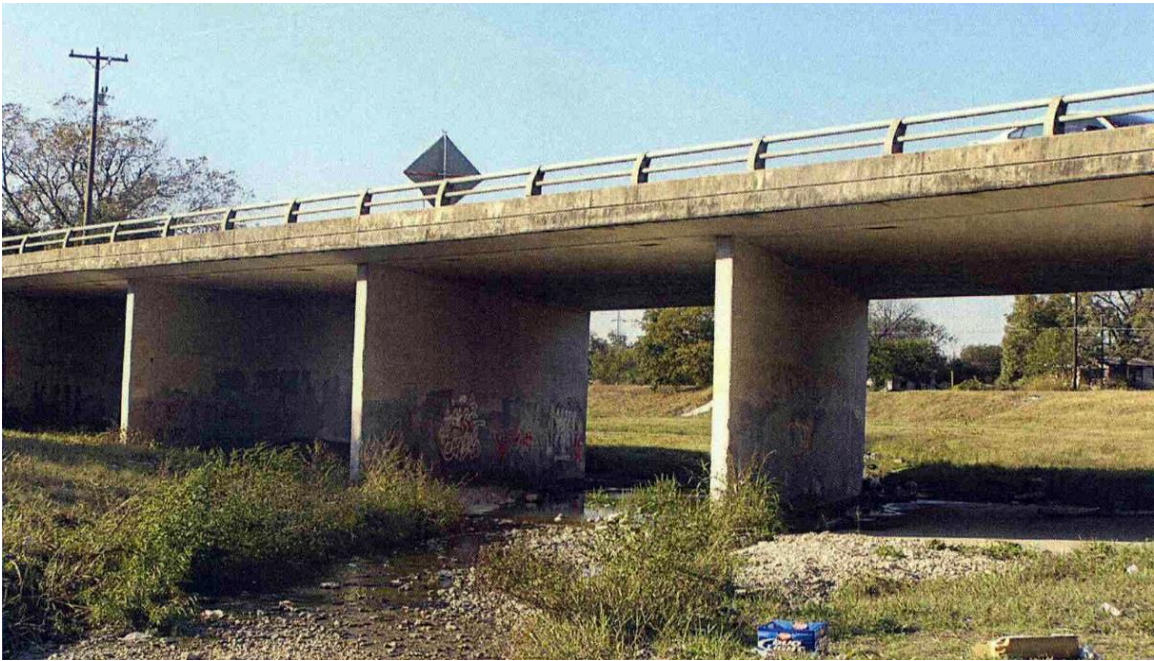
Figure 1. Example of a typical prestressed-concrete slab. Mead & Hunt photograph.
