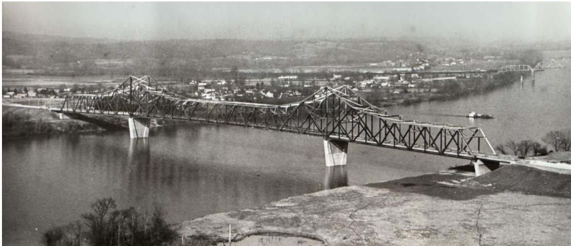
Figure 23. Silver Memorial Bridge (BARS #27A063) shortly after its completion in 1969, photo by the West Virginia Department of Highways. 162
