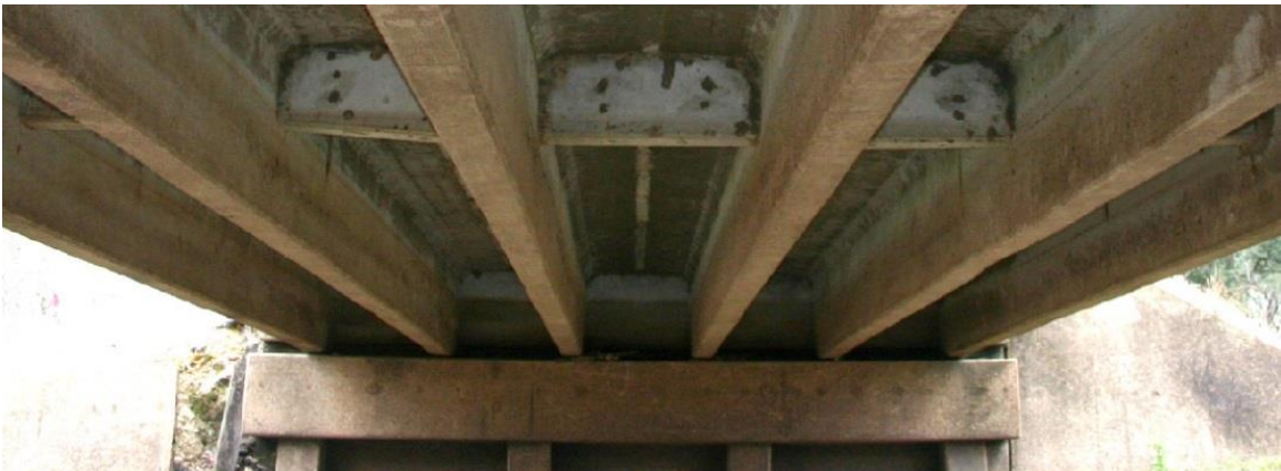
Figure 2. Example of a reinforced-concrete tee-beam structure. Mead & Hunt photograph.
