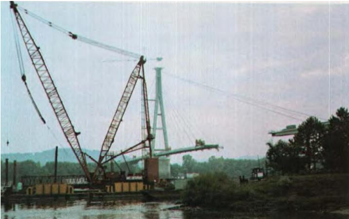
Figure 39. Undated construction image of the East Huntington Bridge (BARS #06A215). 320 Barge cranes were used to construct the deck segments.
