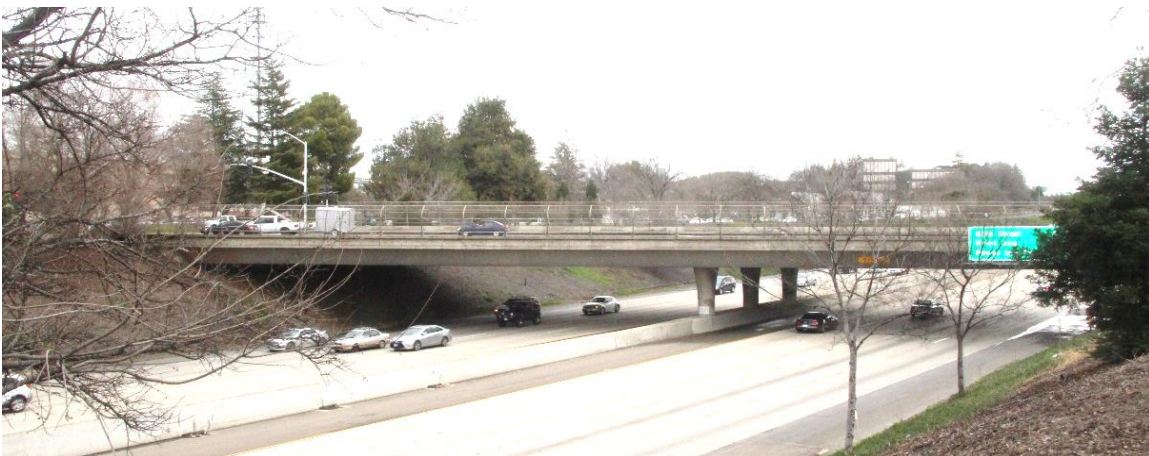
Figure 15. Bridge over Highway 50 in Sacramento, constructed in 1971 with single central pier for improved safety and aesthetics. Mead & Hunt photograph.
