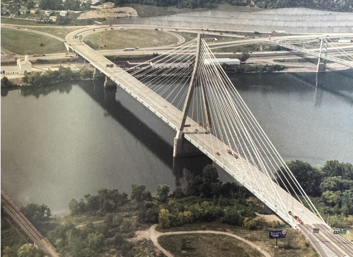
Figure 40. The Veterans Memorial Bridge in Weirton (BARS #05A060), c.1990. 324
