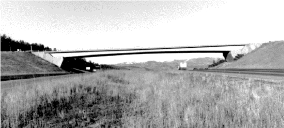
Figure 18. Genesee Park Bridge near Golden, Colorado. 117
