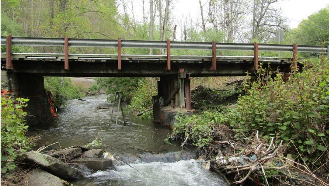
Figure 7. 1965 timber stringer bridge in Raleigh County, West Virginia. 35
