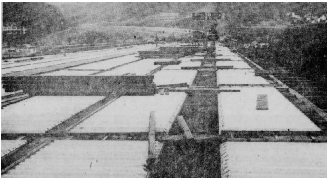
Figure 37. 1976 image of the galvanized steel forms in place on the Jennings Randolph Bridge (BARS #15A025) before the deck was poured. 299 The corrosion-resistant material helps to prolong the life of the deck.
