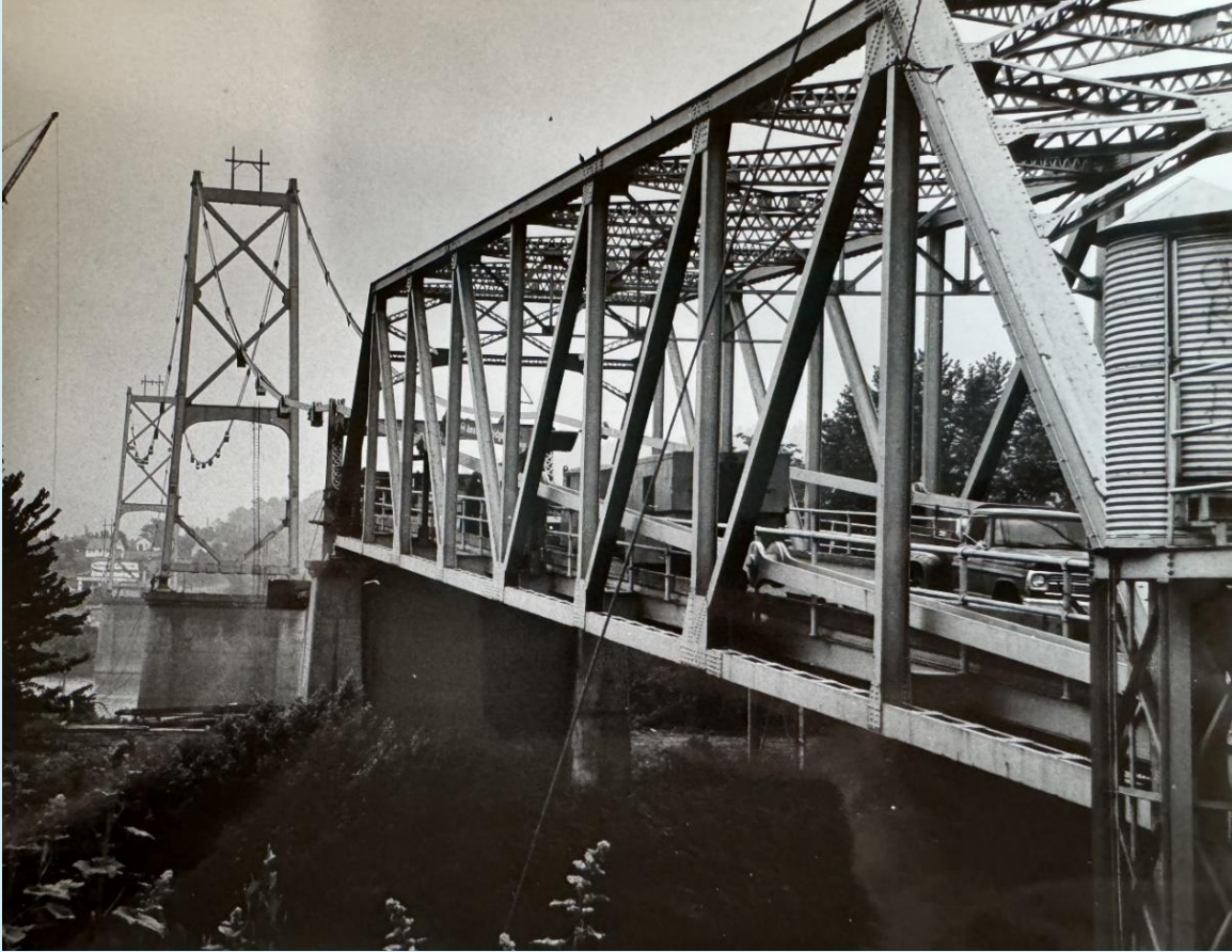
Figure 21. The St. Marys bridge being dismantled in 1971 to make way for its replacement. 140
