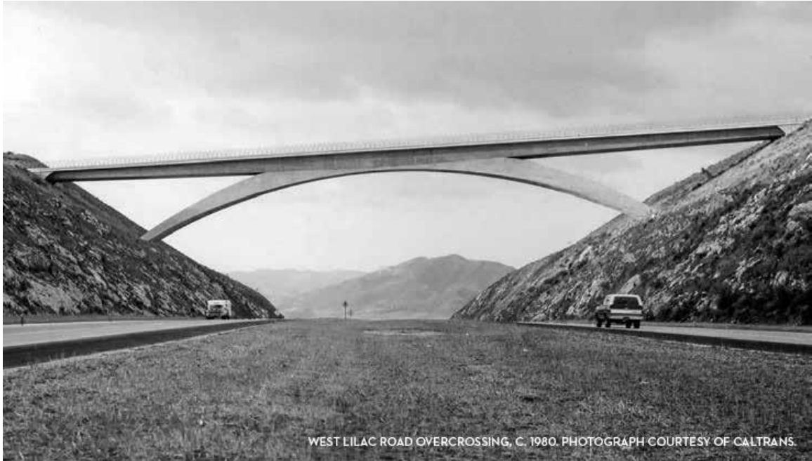
Figure 19. Lilac Road Overcrossing in San Diego County, California, c.1980. Caltrans photograph.
