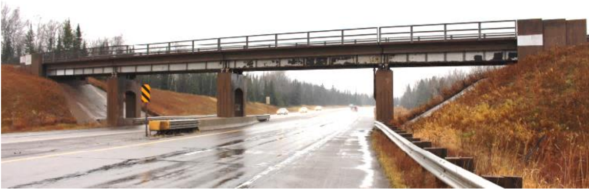
Figure 14. Highway overpass in Minnesota constructed in 1962 with intermediate piers adjacent to travel lane. Mead & Hunt photograph.
