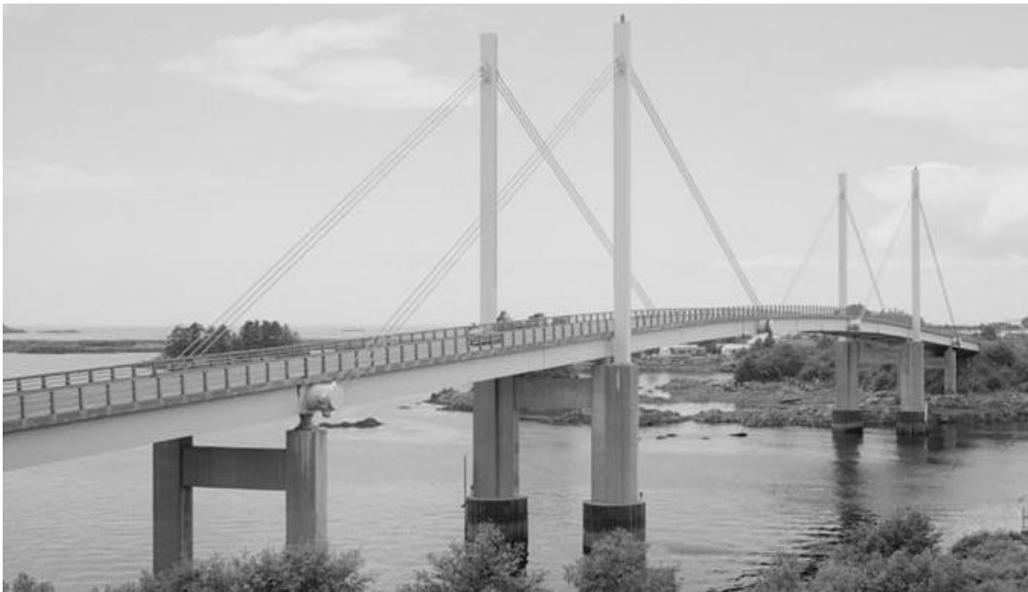
Figure 13. The O'Connell Bridge in Sitka, Alaska, is the first cable-stayed girder bridge constructed in the U.S. 69
