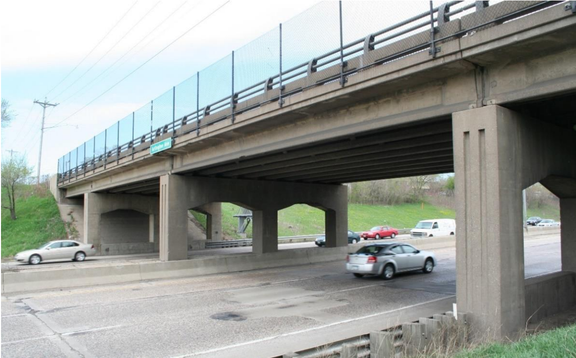
Figure 6. Example of a prestressed-concrete I-beam bridge constructed as part of the new Interstate Highway System. Mead & Hunt photograph.
