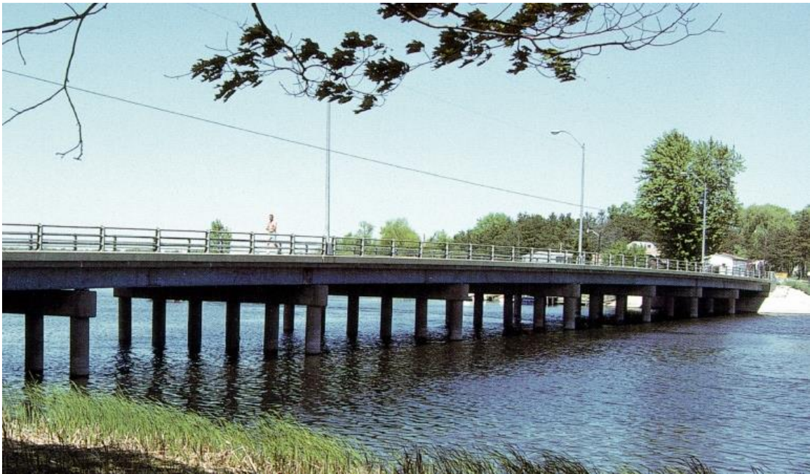
Figure 11. The Stearns Bayou Bridge, built in 1966, was the nation's first documented use of galvanized steel throughout a bridge superstructure. 56
